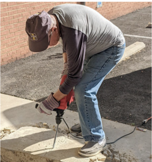
Beware Methodists with jackhammers! Clinton is busting the place up . . . not! He's hard at work breaking the old concrete ramp into pieces so it can be disposed of.
