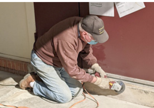
Wilmer is sanding the outer step, preparing it for the new deck and ramp to be built!
