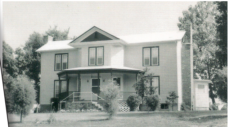
Green farm house "Old Green Building" which was the birthplace of St. Luke's in 1963 stood where the first level of the lower parking lot is today
